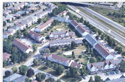
Aerial View of 572 Crystal Drive, known as Sunshine Homes
